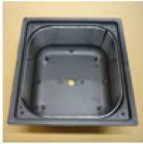
Fig.1 Install 3M Vibration tape to metal surfaces.
